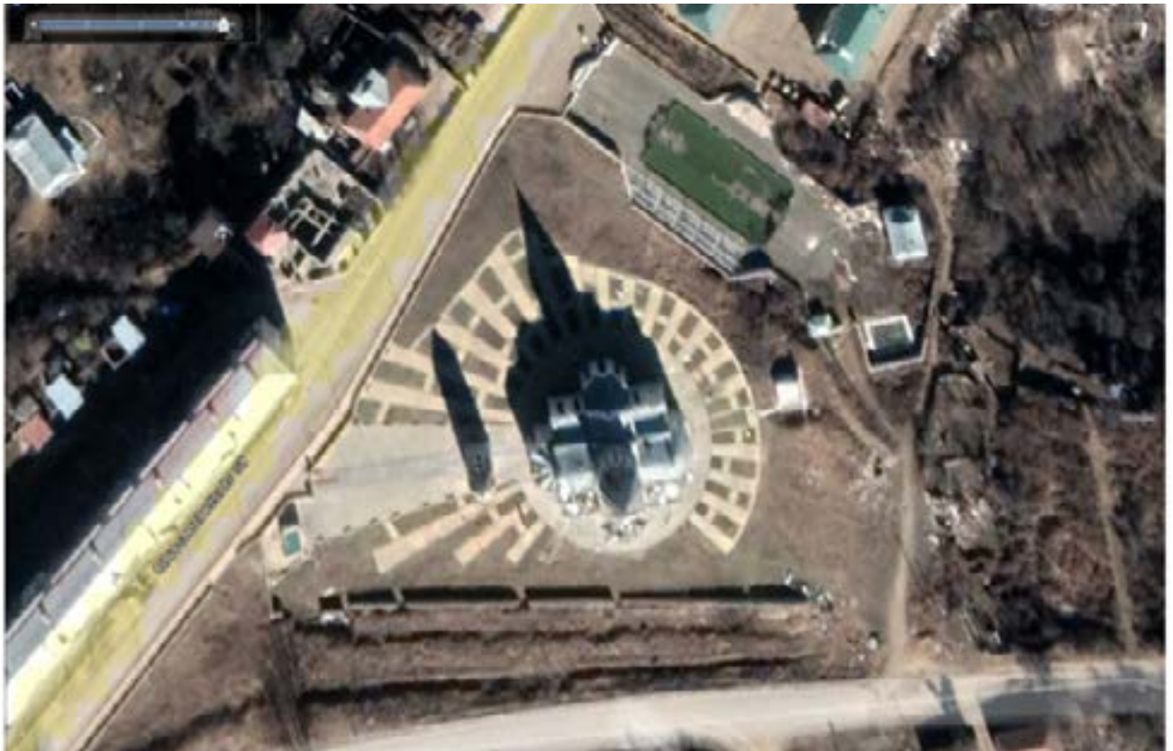
Figure 13.7. Shushi's St. Christ the Savior (Ghazanchetsots) Cathedral after the strike, 15 February 2021 (Source: Google Earth).
