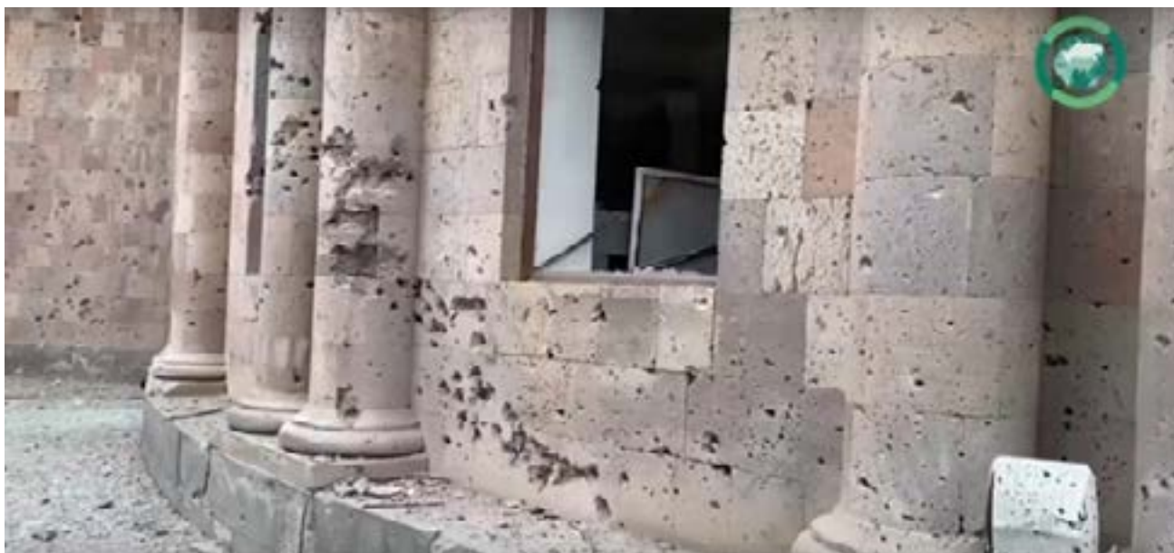
Figure 15.36. Fragmentation damage to buildings at Martuni's municipality, 1 October 2020 (source: Federal News Agency).
