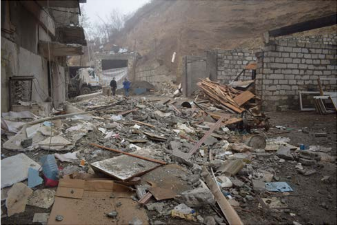
Figure 7.43. 5, Isakov avenue, Stepanakert city (consequences of the shelling on 4 October 2020), 10 December 2021 (Source: Fact-Finding Group).
