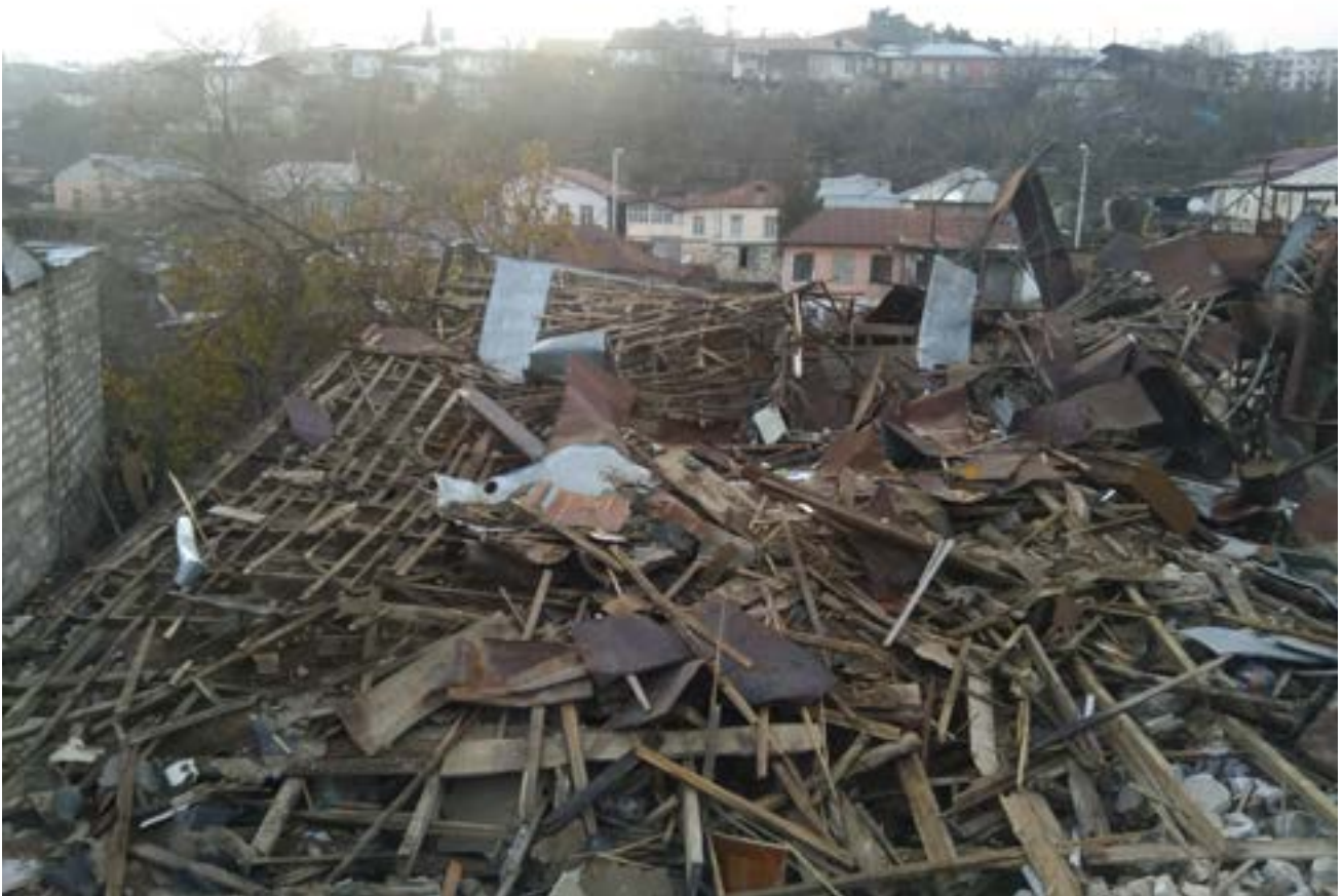
Figure 15.54. Roseta's neighbor's house after attack, 31 October 2021 (Source: Fact-Finding Group).
