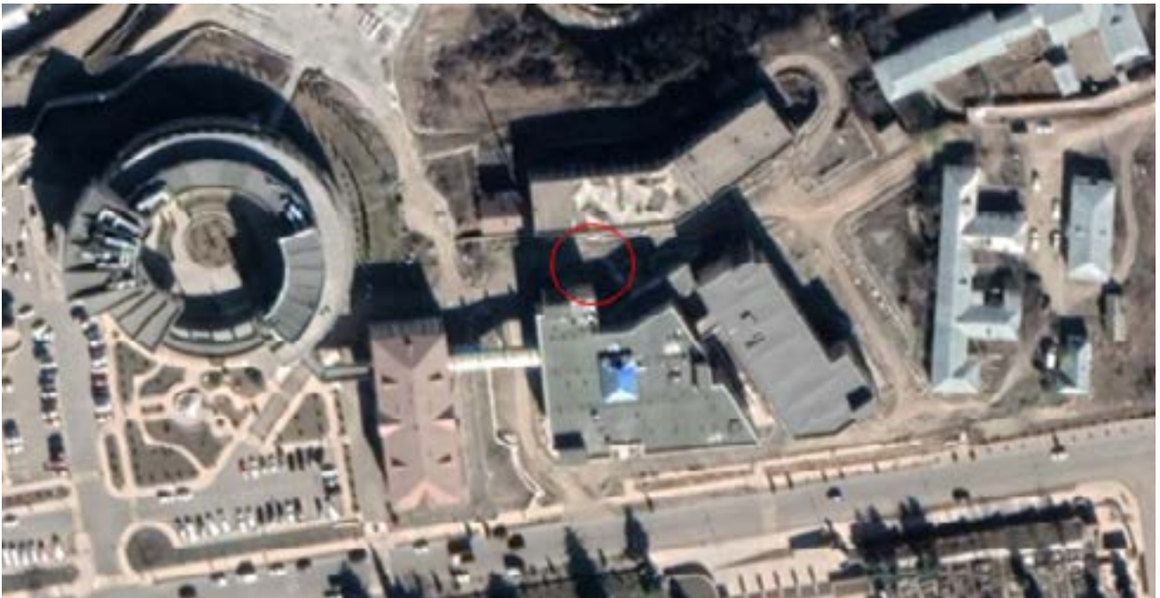
Figure 15.10. Satellite view showing the approximate area of the blast which caused damage to the Maternity Hospital, 28 October 2020 (Source: Google Earth).
