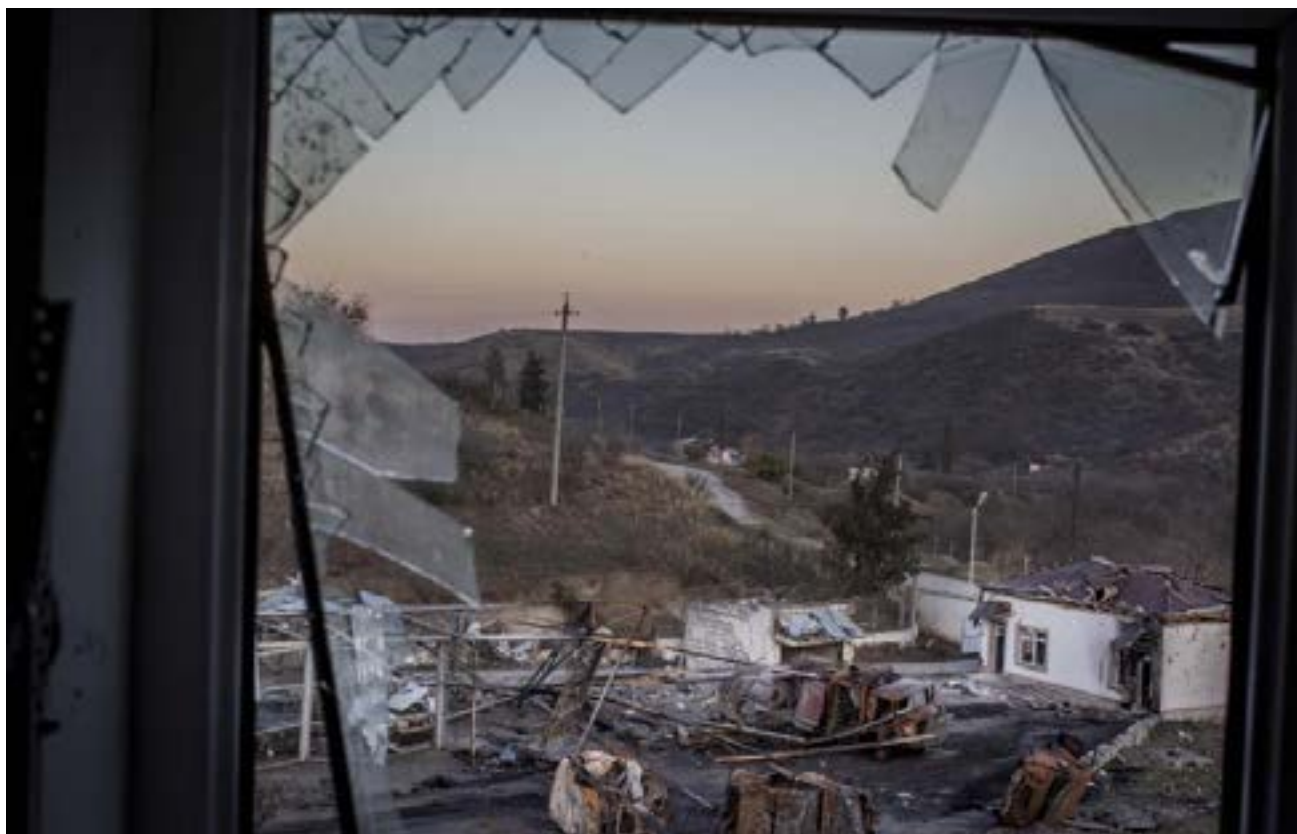
Figure 15.5. Damage to the area of the hospital where the vehicles are held, 14 October 2020. This area was hit directly with a munition as shown in the video evidence (Source: Human Rights Watch).
